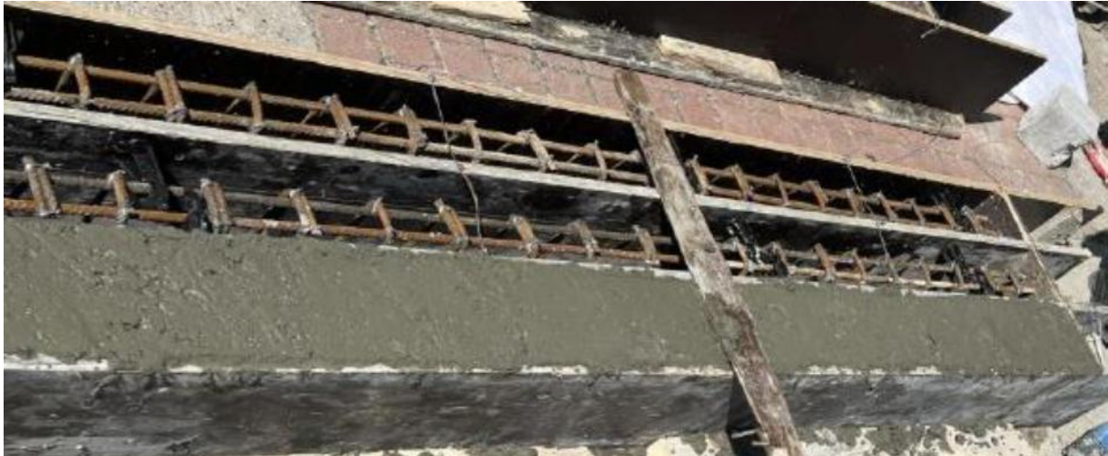
Fig.2. Casting concrete of beams.
